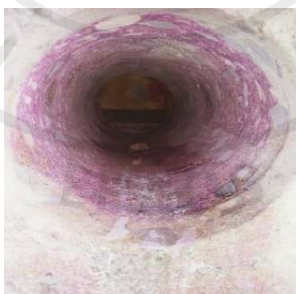
Figure 1: Carbonation Test of The Core
